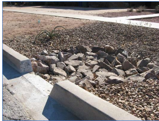
A rock apron protects against soil erosion where curb cuts draw stormwater into bioretention areas.
