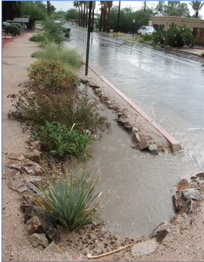
A curb cut draws stormwater from the street into a bioretention basin in the right-of-way.
