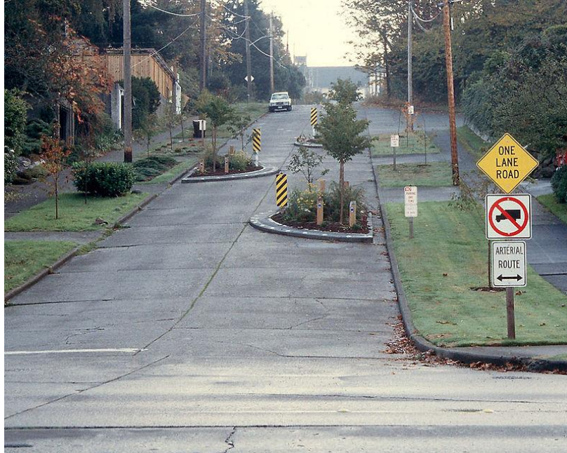
FIGURE 46: EXAMPLE OF A CHICANE (DRDUL, 2006)
