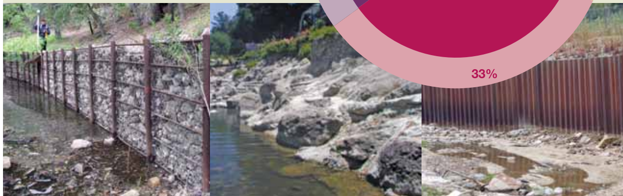
Photos (left to right): Fencing and gabion, concrete boulders, corrugated fencing.
