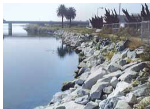
Streambank hardening should only be used as a last resort when bioengineered solutions are not technically feasible.
