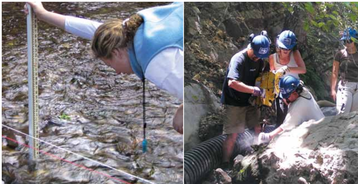
Left: Stream Team member measuring water depth. Right: Barrier removal by jackhammer at Solstice Canyon. Photo credit: Heal the Bay
