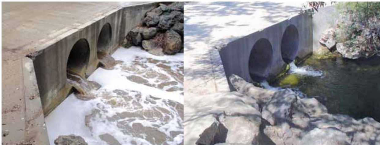
Culvert at Las Virgenes Creek showing high (left) and low (right) turbidity. Photo credit: Heal the Bay
