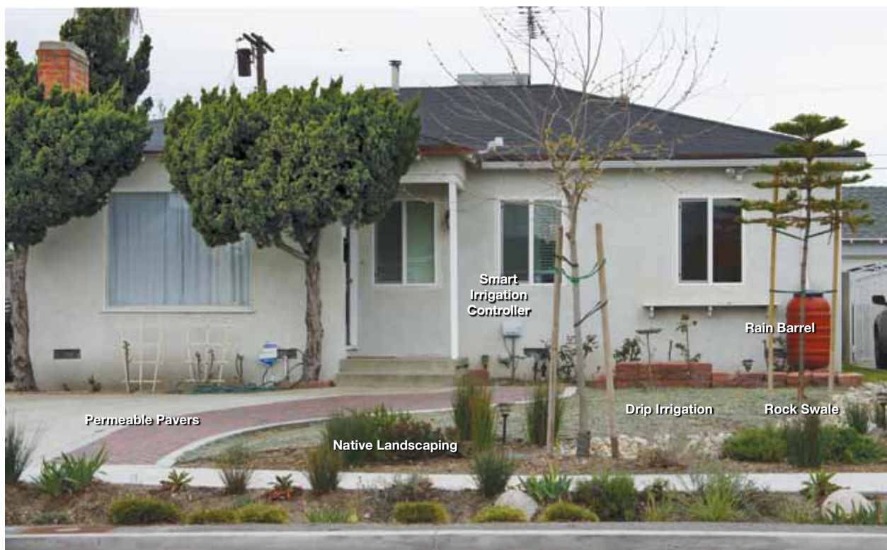
Local governments should adopt Low Impact Development (LID) ordinances that require onsite capture and reuse, or infiltration of 100% of the runoff generated from the 85th percentile storm. Pictured: Elmer Ave. Sun Valley LID demonstration house.
