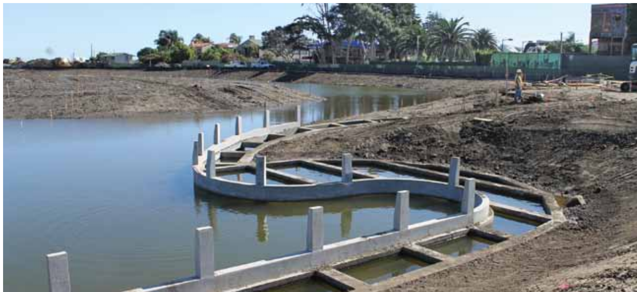
The Malibu Lagoon Restoration and Enhancement Project currently underway will greatly help improve circulation and aquatic habitat conditions. Photo: Heal the Bay
